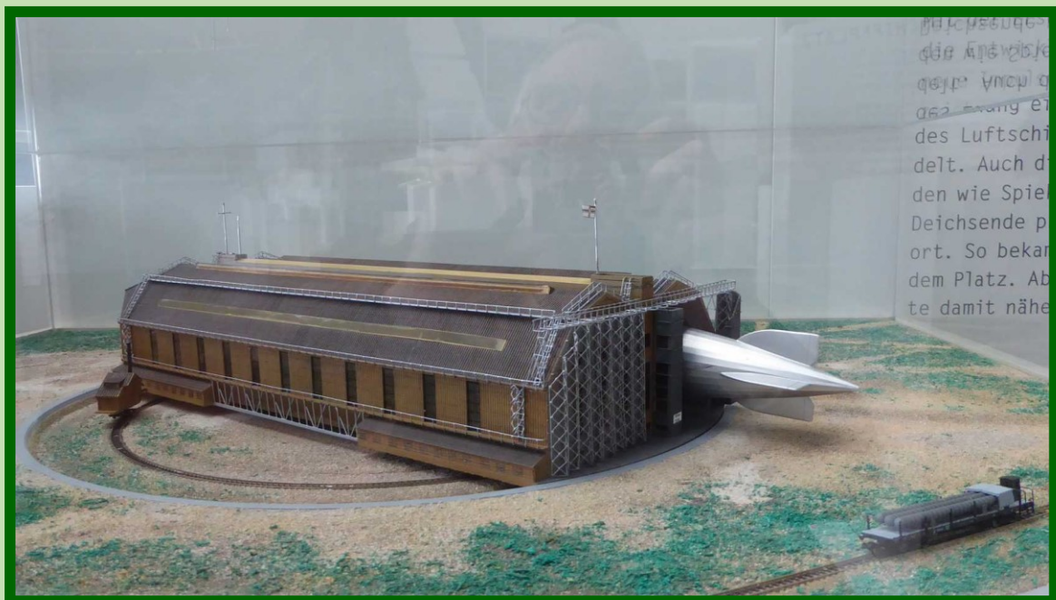
What the aircrews didn't see – the Drehhalle (rotating hanger) at Nordholz, which could turn through 360°, to mitigate the effects of crosswinds when moving the airships in or out. This was to avoid hitting the fragile airship on the hanger doors. A complete rotation took an hour.
